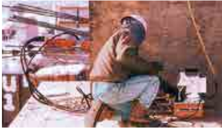
The PE60 used for pre-stressing.
